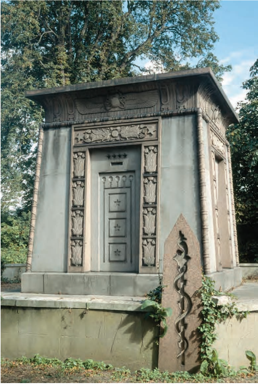
Plate xxix Mausoleum of the 2nd Earl of Kilmorey (1787–1880) and his mistress, Priscilla Hoste (died 1854). It was originally erected to designs by Henry Edward Kendall the Younger (1805–85) in Brompton Cemetery, London, in 1854, was moved to Woburn Park, Chertsey, in 1862, and then translated to Gordon House, Isleworth, Middlesex, in 1870 (MaCh A240902).
